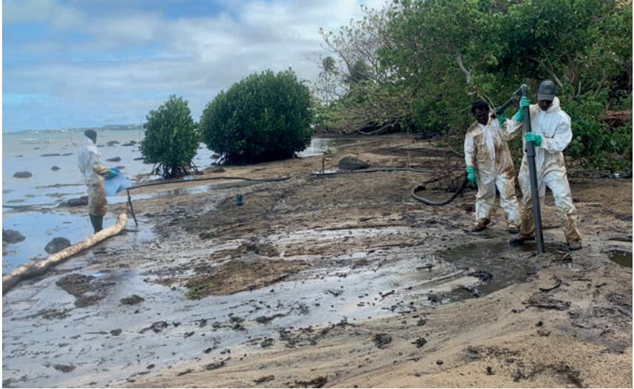
Flushing oil from substrate, Mauritius
