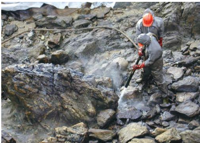
▲ Figure 17: Low-pressure water is used to flush oil from between rocks, to be collected by sorbent material further down the shoreline.
