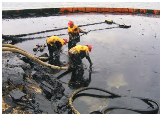
▲ Figure 3: Recovery of fluid bulk oil from the shoreline using a rope mop skimmer and vacuum pumps.
