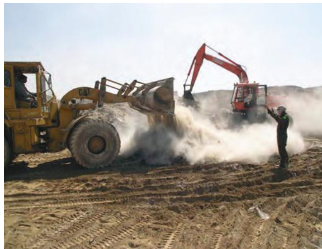
▲ Figure 18: Stabilisation of oily waste using quicklime.
