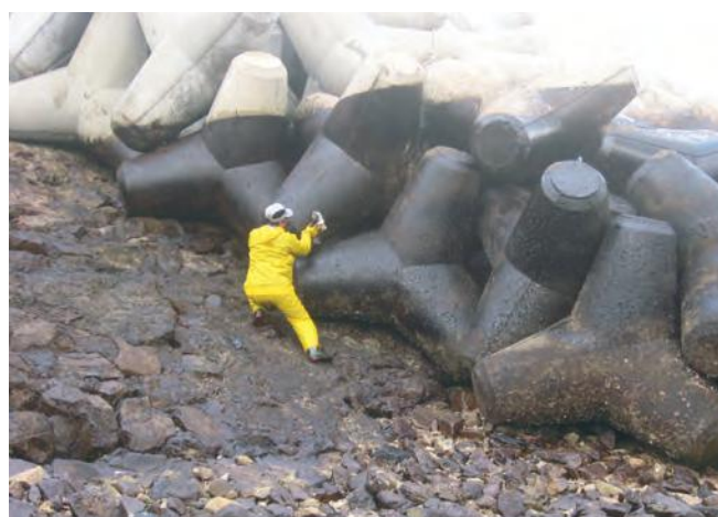
▲ Figure 33: Cleaning of oiled tetrapods is problematic, as oil within the structure is difficult to reach.
