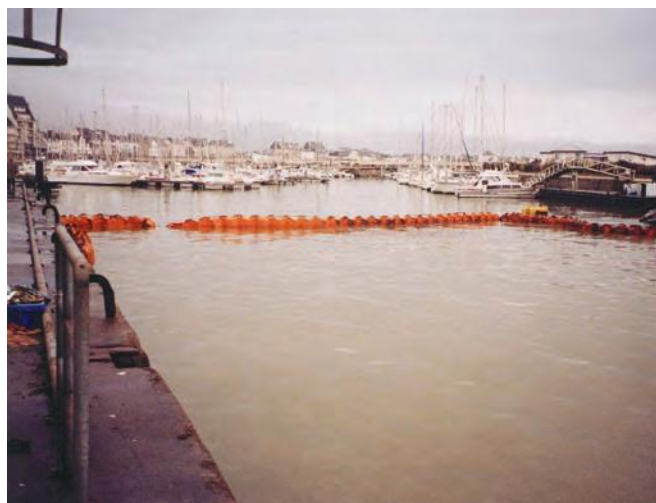
▲ Figure 2: Successful booming of marina entrances can be compromised if the boom is damaged by vessels entering or leaving.
