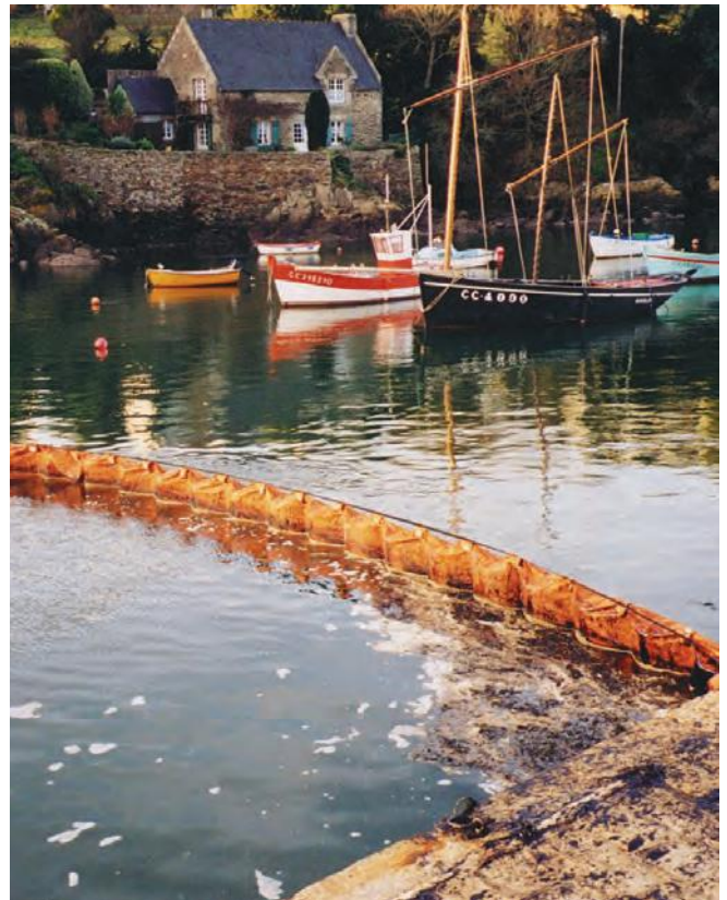
▲ Figure 1: Fence boom deflecting oil from moorings.
