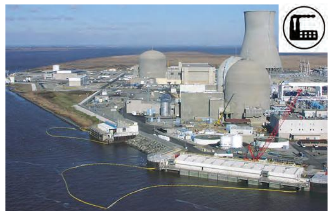
Figure 6: Power station with a water intake in the foreground. Several deflection booms are deployed to prevent the ingress of oil.
