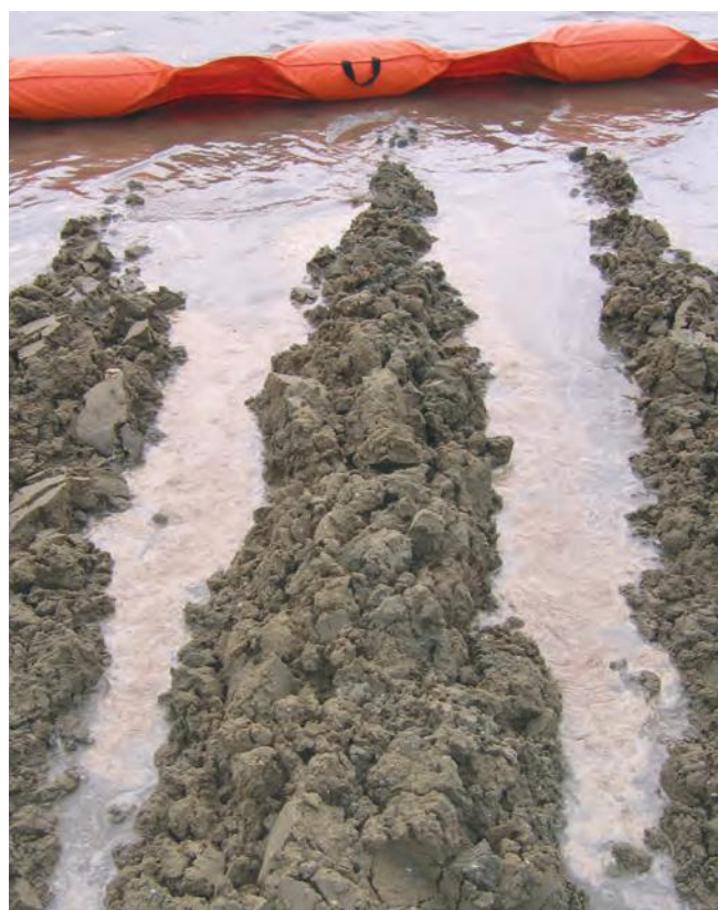
▲ Figure 25: Contaminated beach substrate is brought to the surface by ploughing. Oil is then released on the incoming tide for collection at the water's edge.
