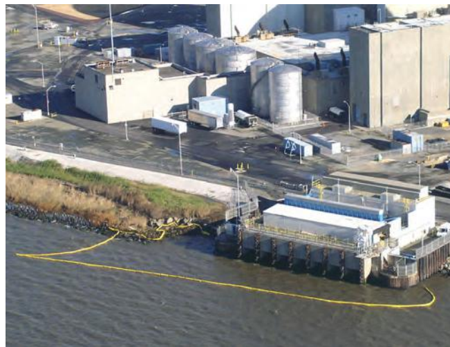
▲ Figure 13: Curtain boom deployed in front of a power station cooling-water intake.
