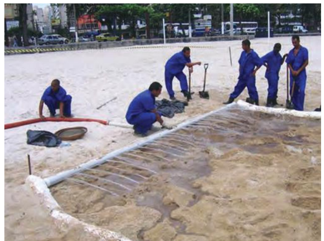
▲ Figure 1: Cleaning of oiled sand in-situ by low pressure flushing, with sorbent boom deployed appropriately to capture released oil.
