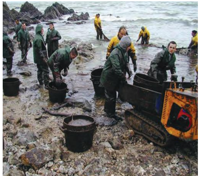
▲ Figure 1: Manual removal of bulk oil. The use of manpower for the selective recovery of oil from a shoreline minimises the amount of clean material removed.
