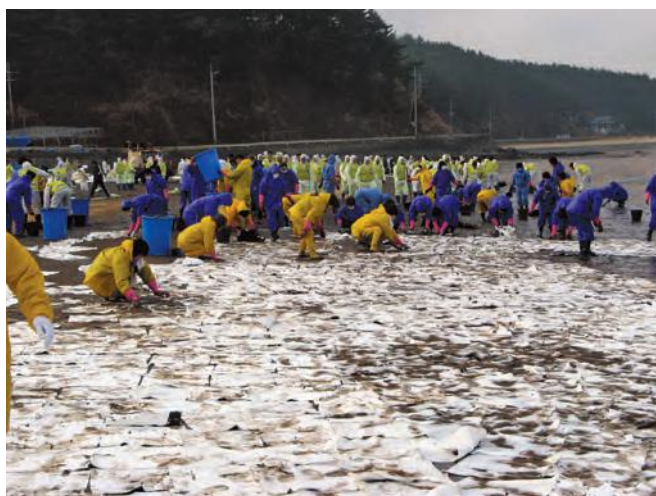
▲ Figure 9: The large-scale use of sorbent to recover oil on a hard sand beach. The use of sorbent material should be appropriate to the scale of contamination, bring an appreciable benefit to the response and not unduly add to the waste requiring disposal.
