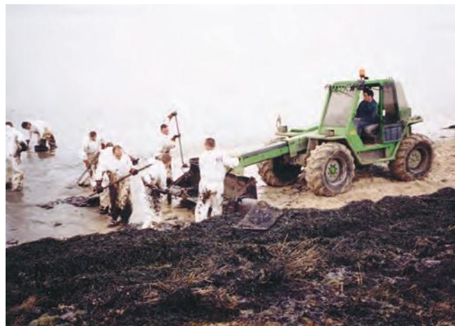
▲ Figure 8: Manual removal of oil and oiled seaweed into a telescopic bucket. This method allows oiled material to be selected in preference to clean material, minimising the amount of waste.
