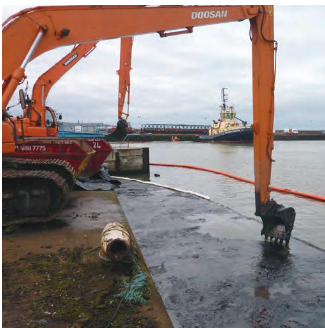
▲ Figure 5: Civil engineering machinery employed to recover oil from a port area. In this situation, the water temperature was below the pour point of the oil, causing the oil to become semi-solid, precluding the use of skimmers.
