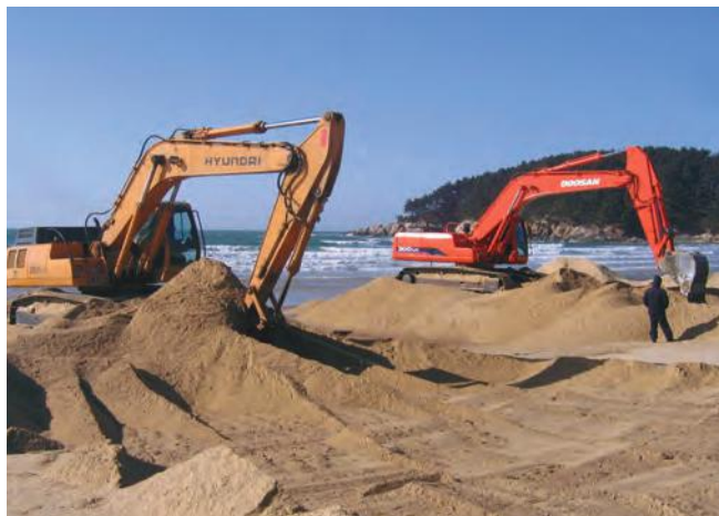
▲ Figure 18: Lightly contaminated sand is moved to the intertidal surf zone for washing on subsequent tides.
