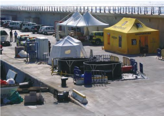
▲ Figure 45: Temporary buildings sited close to a work site provide catering and sanitary facilities for the workers.
