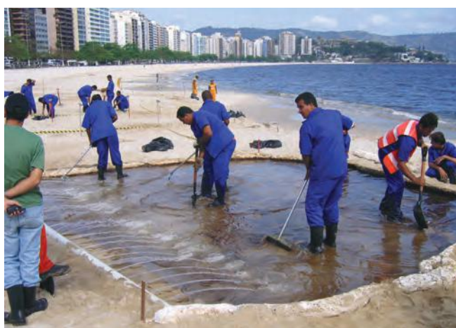
▲ Figure 16: Oil buried in a sand beach is flushed out using low pressure water supplied through lances and perforated pipes. The substrate is also agitated manually to encourage the oil to separate from the sand. The oil is then recovered by the sorbent boom surrounding the work area.
