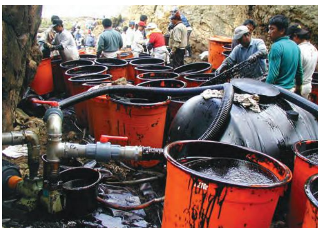
▲ Figure 13: Oil collected on a rocky shoreline temporarily stored in large open-topped bins. Pumps were required to transfer this oil to the top of the cliff and then to road tankers.
