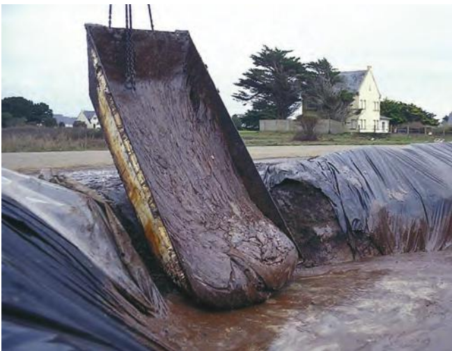
▲ Figure 11: Skip emptying emulsified fuel oil into a lined temporary storage pit.
