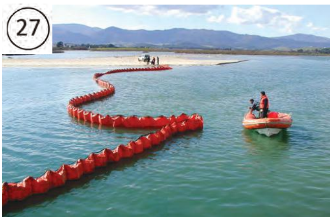
Figure 5: Boom deployment site near the river mouth. The boom is being set to deflect oil to a collection point with good access on the shore.
