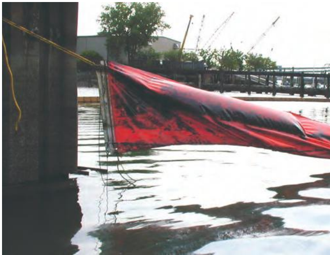
▲ Figure 16: Use of an insufficiently long mooring line has caused the boom to become suspended at low tide, allowing oil to pass beneath. Regular adjustment of lines would be required to maintain the boom in an effective position throughout the tidal cycle. Sliding moorings would be more effective in this scenario.
