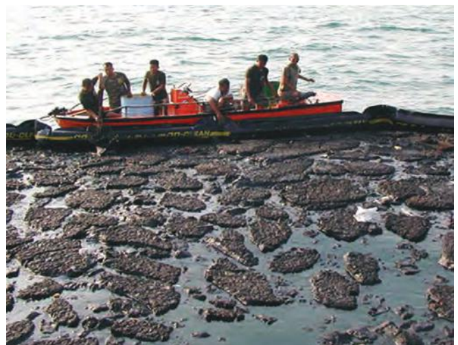
▲ Figure 6: Semi-solid oil contained within a boom. The difficulties of pumping the oil can limit the available disposal routes.
