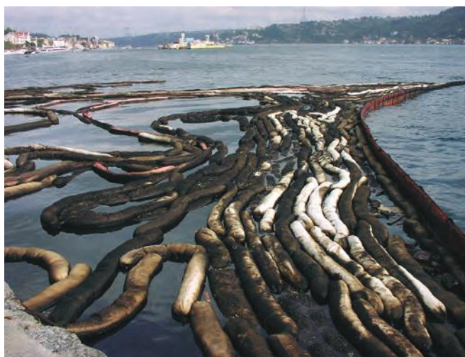
▲ Figure 7: Partially oiled sorbent boom. The large-scale use of sorbent materials should be avoided in order to minimise waste generation.
