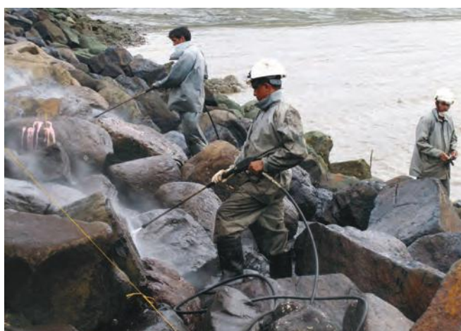
▲ Figure 32: Cleaning of rip-rap using high pressure washers.
