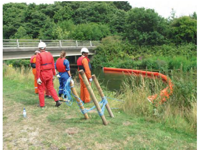
▲ Figure 17: Mooring stakes to hold boom in place on shoreline without trees or other natural anchors.
