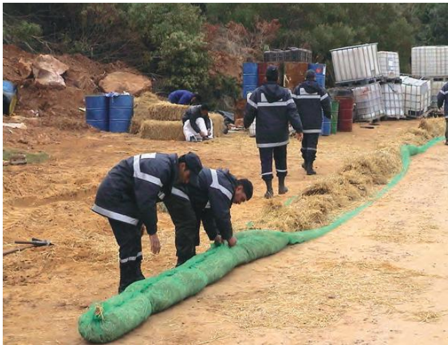
▲ Figure 20: Improved boom constructed from netting and straw. While not expected to survive more than one tidal cycle, this may nevertheless serve to reduce contamination of the shoreline from incoming floating oil.
