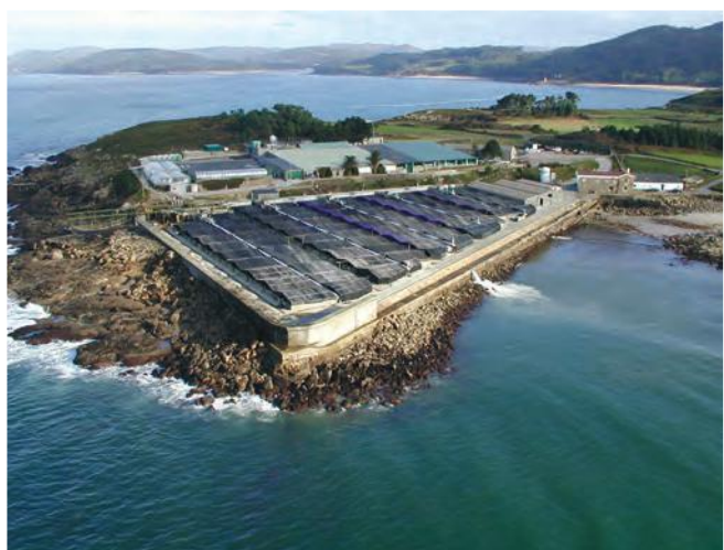
▲ Figure 7: Onshore fish hatcheries require large volumes of clean sea water. Water intakes are usually located below the water surface and may be affected by dispersed oil.
