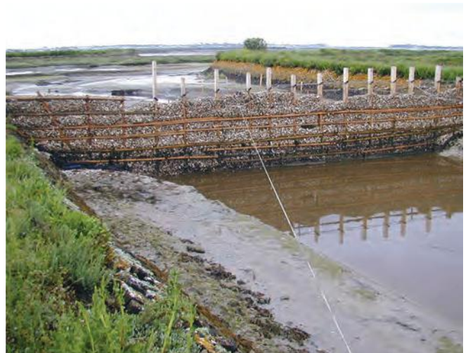
▲ Figure 21: Barrier constructed from oyster-shells, held in place by stakes and nets.
