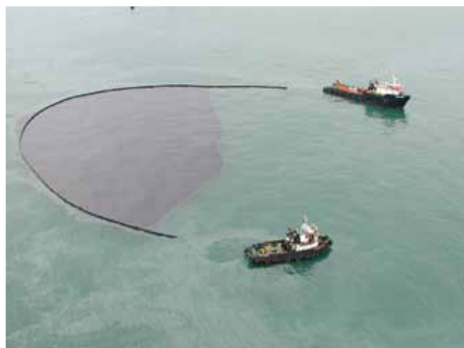
▲ Figure 5: While oil has been contained successfully, these efforts may be in vain without a means of recovery from the water surface and temporary storage of the oil.
