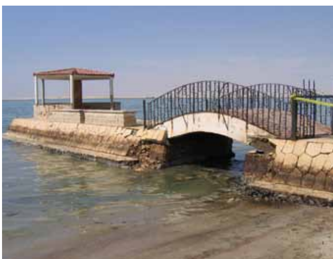
▲ Figure 14: Light oil staining of a stone jetty. This may be easily confused with algae growth.
