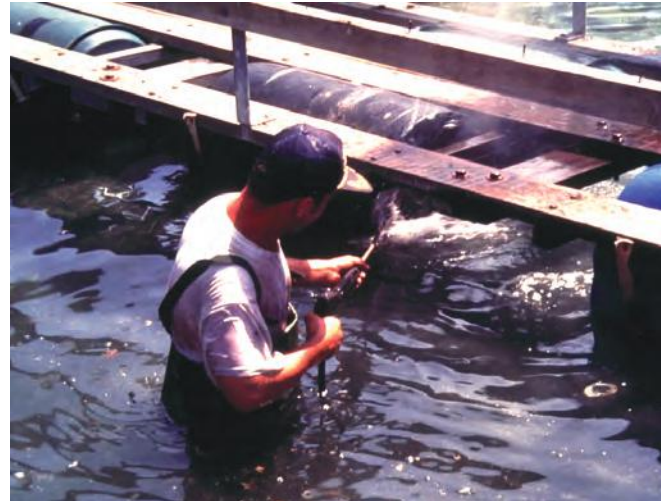
▲ Figure 11: Mariculture facilities can be cleaned in-situ by pressure washing.
