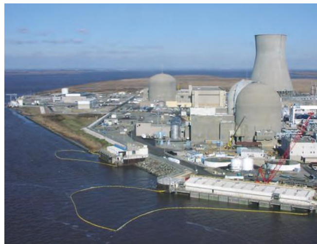
▲ Figure 7: Water intakes should be protected to prevent oil affecting heat exchangers that can be difficult to clean and may lead to the shut down of facilities.
