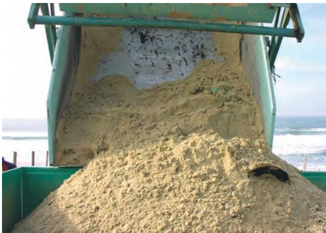
▲ Figure 7: Collection directly by heavy machinery has resulted in a high proportion of clean material and very low concentrations of oil in the waste.
